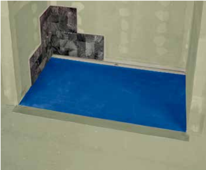
4. Finishing – Natural stone, glass, porcelain, or ceramic tile are applied to the walls and shower base.
