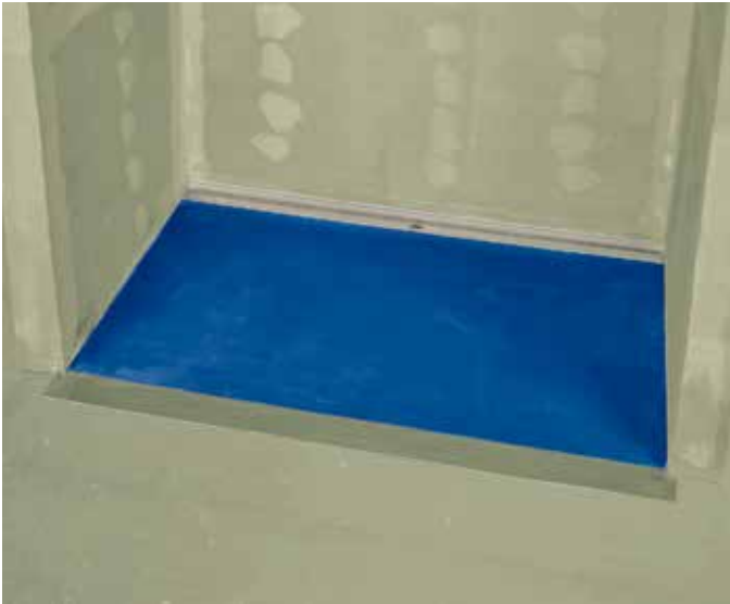
3. Walls and Waterproofing – Appropriate backerboard is mounted to the framing and seated on the flange of the shower base. Liquid or fabric waterproofing is applied over the backer board down to the shower base.
